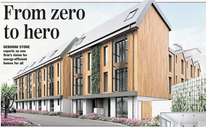
FOSSIL FUEL-FREE: Hilgrove Mews homes have solar panels integrated in the roof, super-insulation and triple glazing to keep them warm
